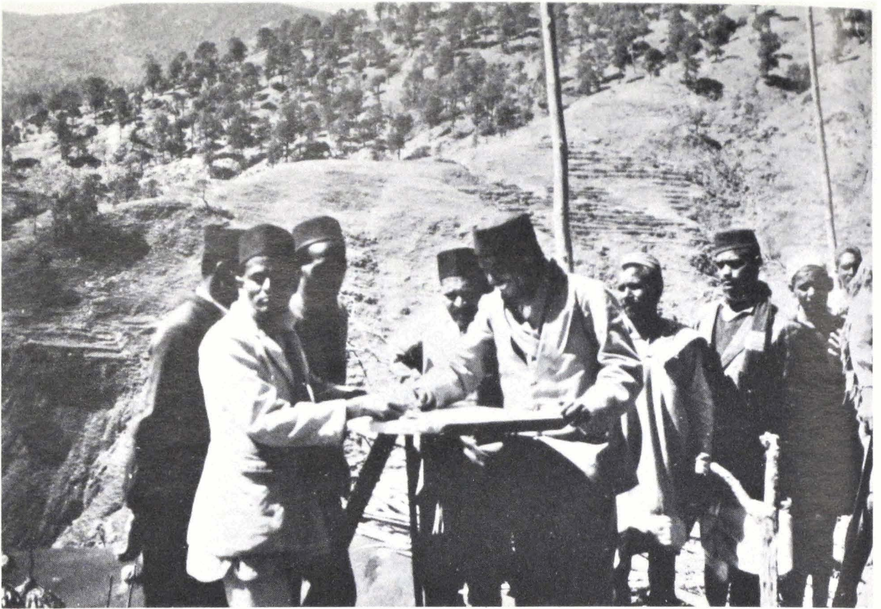
A survey party in the field making maps. With the simplest instruments, they achieved astonishingly accurate results, mapping the fields to a scale of 32" to the mile.
